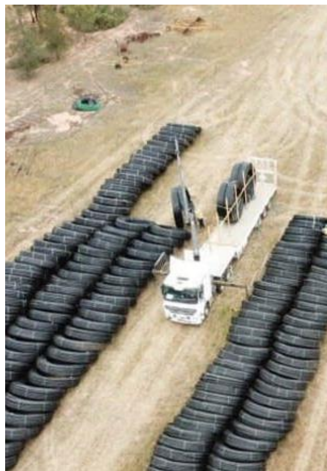
Plastic piping being prepared for installation on the Mitiamo project.
