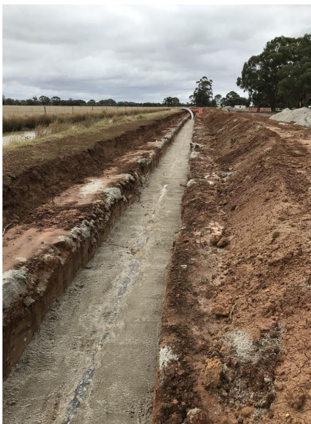
Installation of new 1.2km RO 3A/14 Principal Pipeline (DN710 & DN630)
